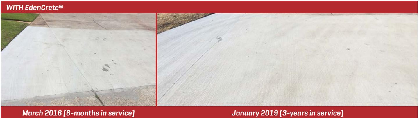
The EdenCrete® surface is still intact with minimal degradation. Within 1-year of placement, the Control was abraded, cracked, and stained.
