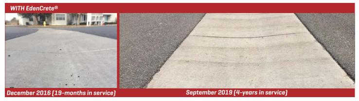
The EdenCrete® surface is still intact with minimal degradation. Reference was abraded, pitted, and scaled within 1-year of placement.
